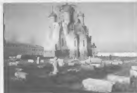
Fig. 14.28. The Louzhetskiy Monastery in Mozhaysk. We see the courtyard. In 1999, some two metres of the turf were removed. The former level of soil can be judged by the dark strip at the bottom of the monastery's cathedral. One can also see that the windows of the cathedral have been elevated except for one window, which had been at ground level when the excavations were conducted. In the foreground we see a few sarcophagi of the XVII-XIX century, unearthed during excavations and arranged in accurate rows. The level of soil in the courtyard now corresponds to that of the XVII century. Photograph taken in 2000.
